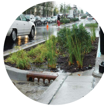
Stormwater Planter w/ Constructed Weirs
