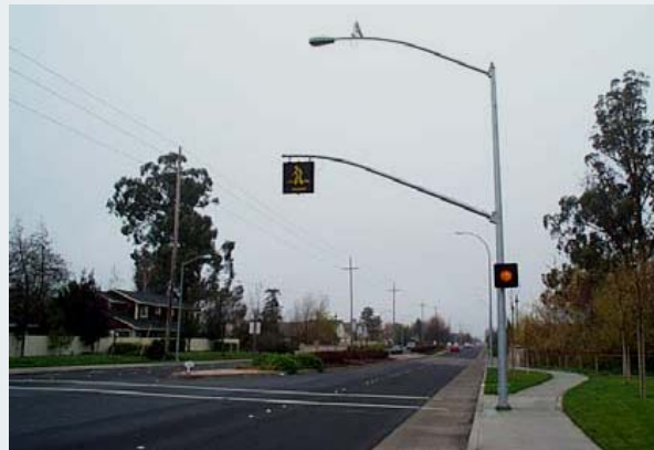
OVER-HEAD SIGNS / LIGHTS
