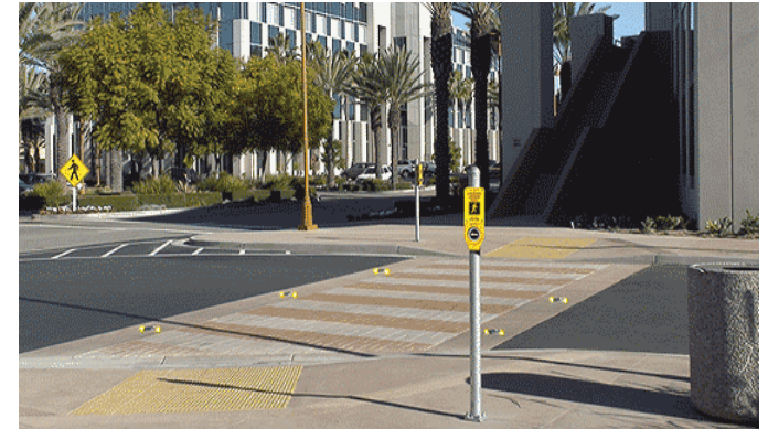
IN-PAVEMENT LIGHTS – PEDESTRIAN ACTIVATED
